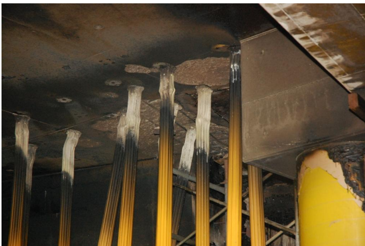
Photo 45 showing basement level one aluminium support props.
