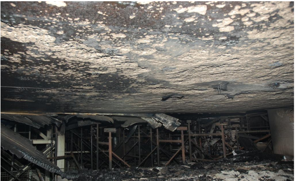
Photo 16 showing Basement level one: Soot deposits to concrete and spalling.
