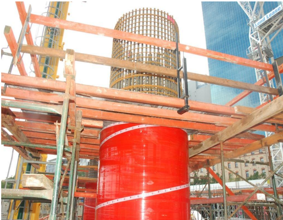
Photo 73 showing an example of the polystyrene product used to form the concrete columns. This picture is taken from a separate area of the Barangaroo site. It is confirmed by Lend Lease staff as being the same as the product used in the fire involved area.
