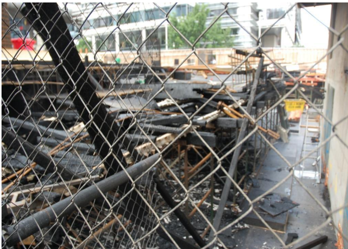
Photo 84 showing fire damage to formwork at ground level. Area inaccessible.
