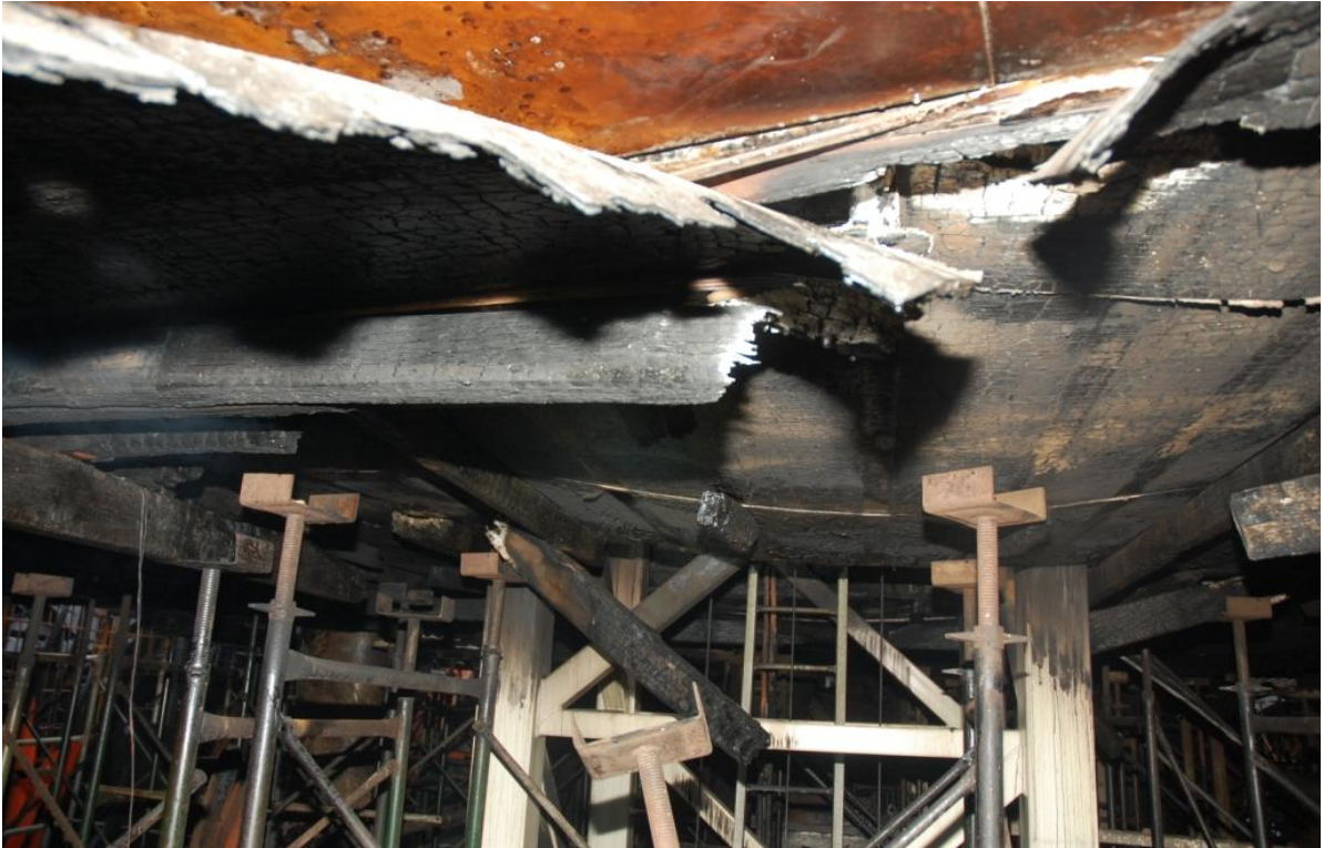
Photo 22 showing Basement level one: Damage at ceiling height.
