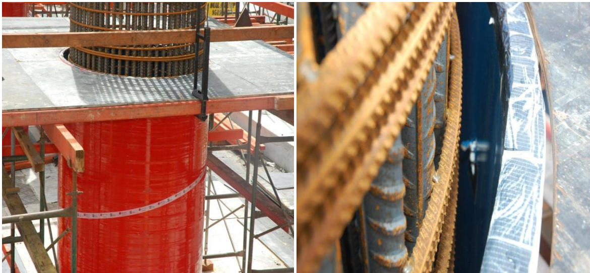
Photos showing the expanded polystyrene foam formwork in use at Barangaroo.
