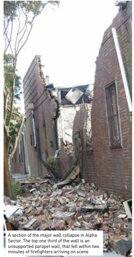
A section of the major wall collapse in Alpha Sector. The top one third of the wall is an unsupported parapet wall, that fell within two minutes of firefighters arriving on scene
