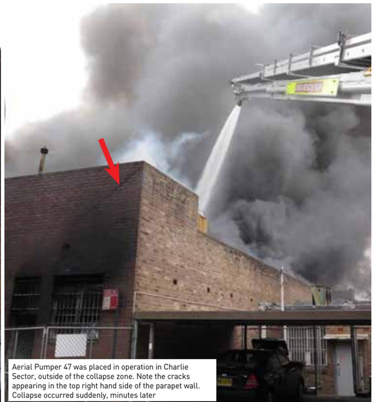
Aerial Pumper 47 was placed in operation in Charlie Sector, outside of the collapse zone. Note the cracks appearing in the top right hand side of the parapet wall. Collapse occurred suddenly, minutes later
