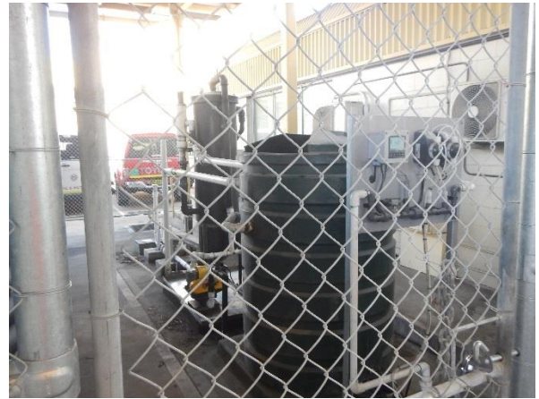
▲ Photograph 14: The interceptor for the site where the internal drains go to.
