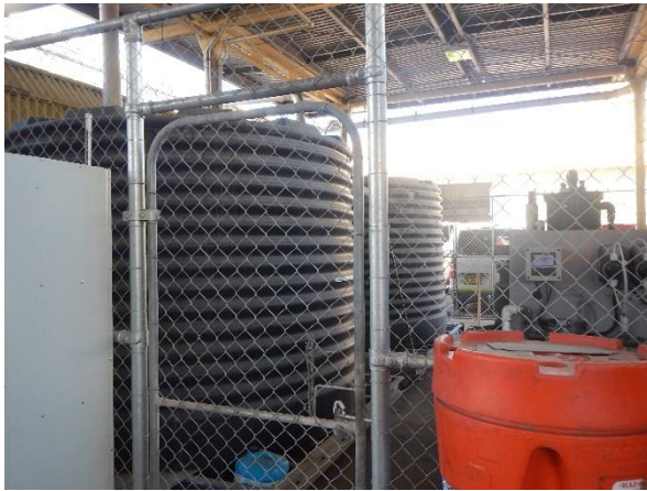
▲ Photograph 13: The interceptor and rain tanks located near the truck wash in the eastern area of the site.
