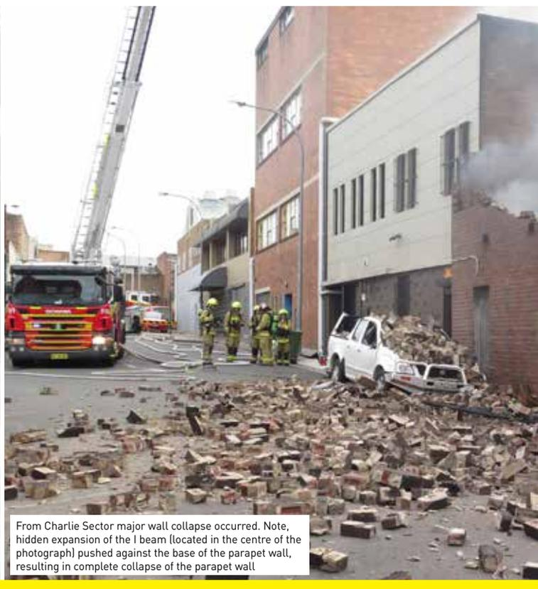
From Charlie Sector major wall collapse occurred. Note, hidden expansion of the I beam (located in the centre of the photograph) pushed against the base of the parapet wall, resulting in complete collapse of the parapet wall
